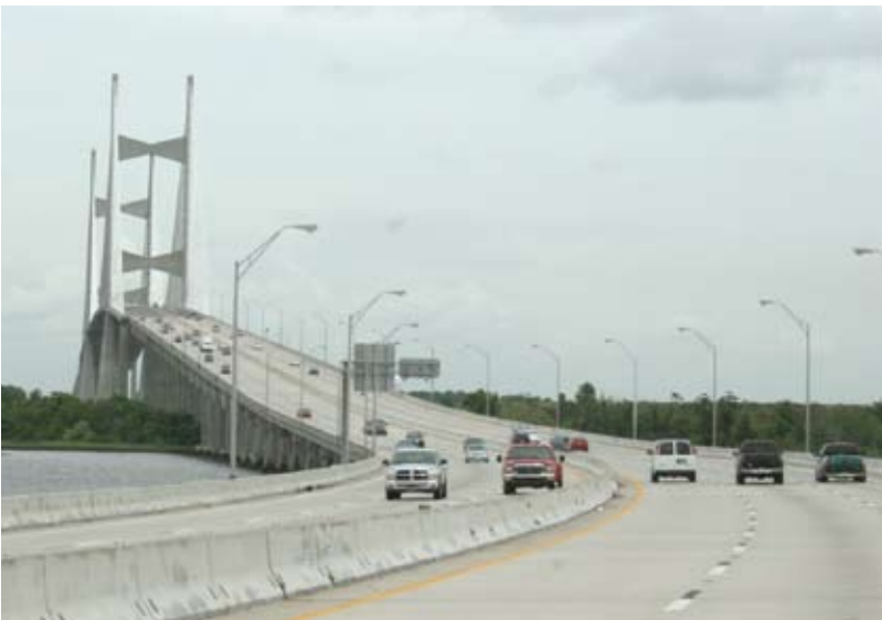
Dames Point Bridge
